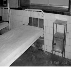
MM4 - Before Renovation June 27, 2005
