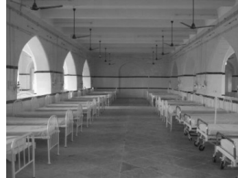
Postop Ward - After Renovation
